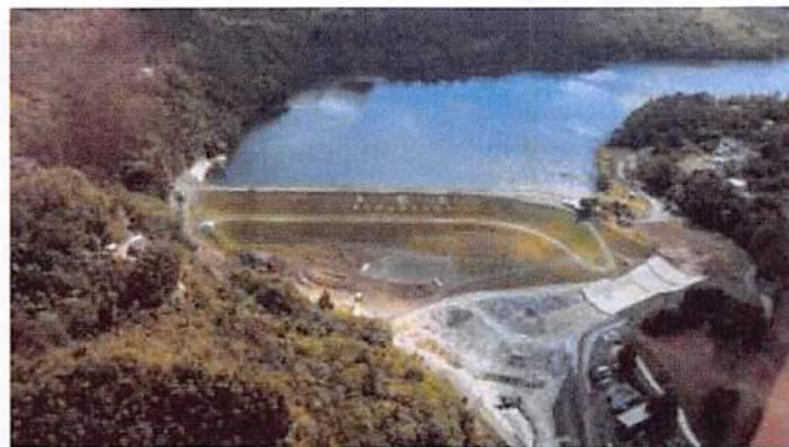
Guajataca Dam after repairs in 2020
