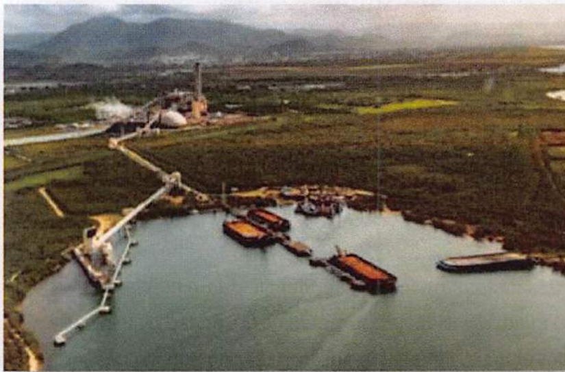
AES Coal Power Plant in Guayama
