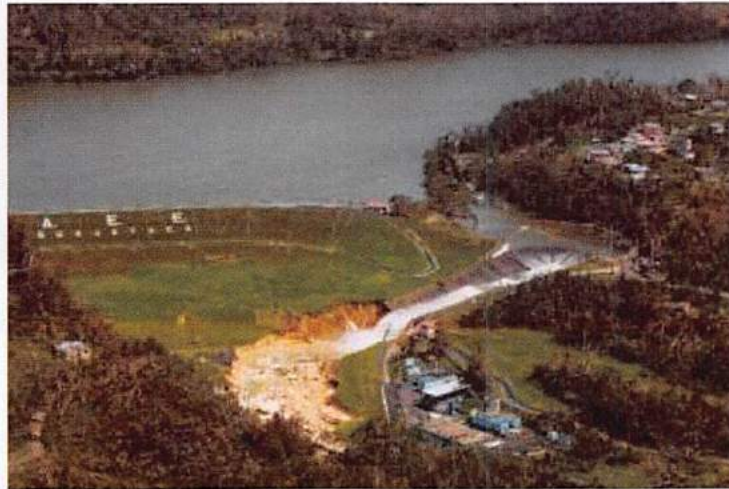
Guajataca Dam failure during Hurricane Maria 2017
