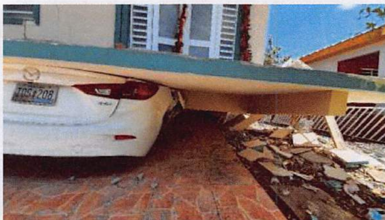
Houses on stilts or columns fell directly to the ground
