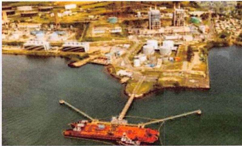
Aguirre and Aguirre Combined Cycle Power Plant
