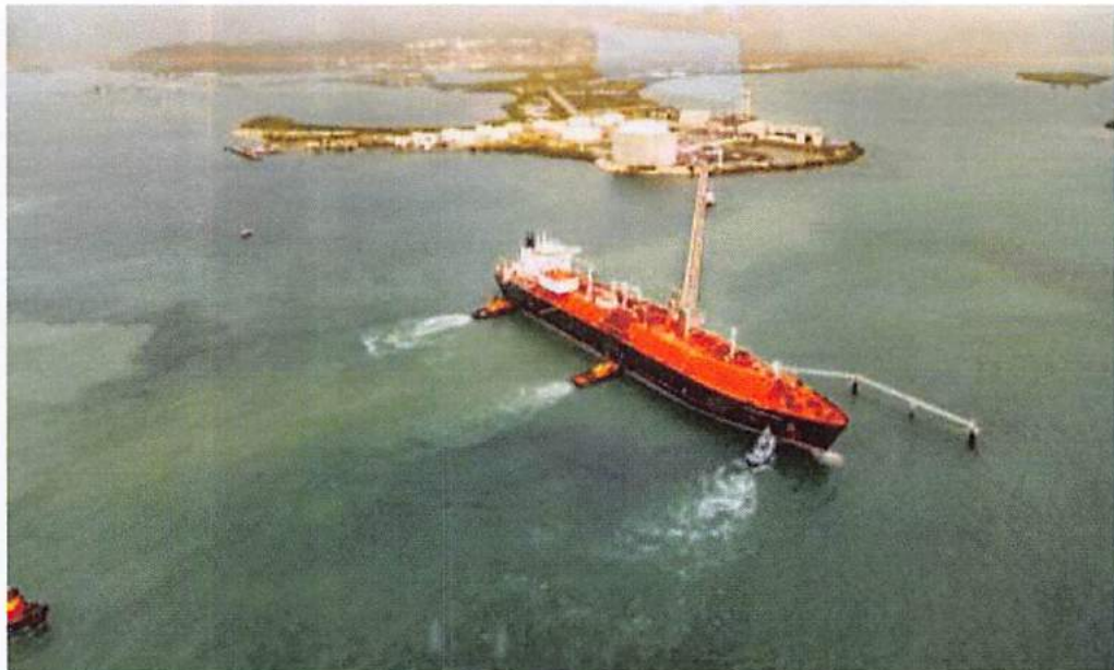
Liquefied Natural Gas Terminal of Eco Electrica
