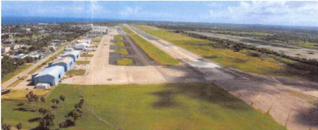
Rafael Hernandez Airport (BQN) Aguadilla Runway 8/26: 11,702ft.
