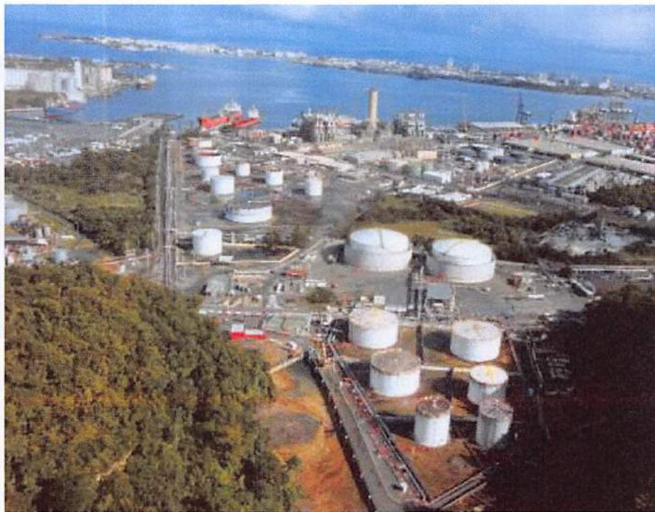
Total Petroleum fuel transfer pipeline: .68 miles
