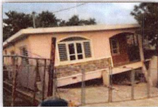
Stilt houses in Guánica that collapsed during the earthquake of January 7, 2020
