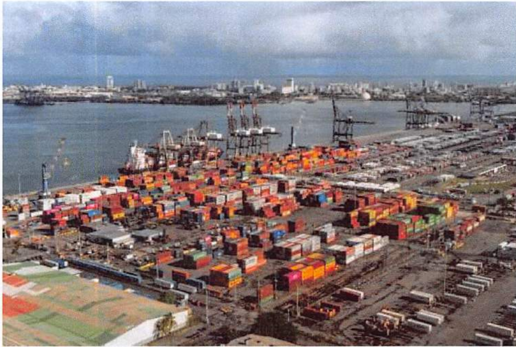
Container storage and distribution area in the San Juan Port
