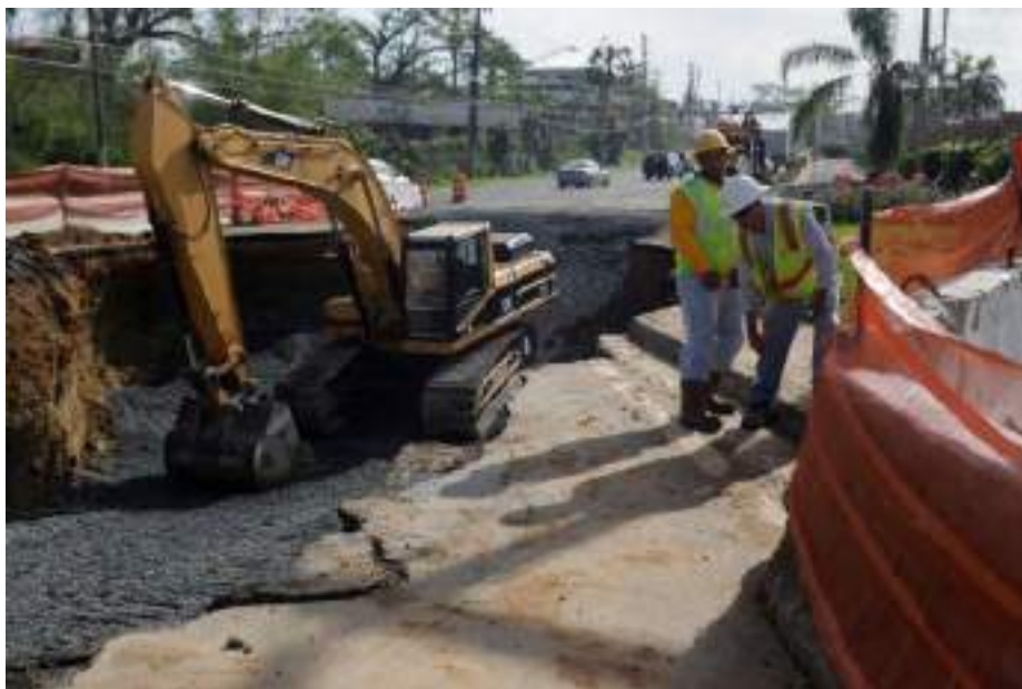
Figure 248: Rebuilding a Sinkhole after Hurricane Maria
