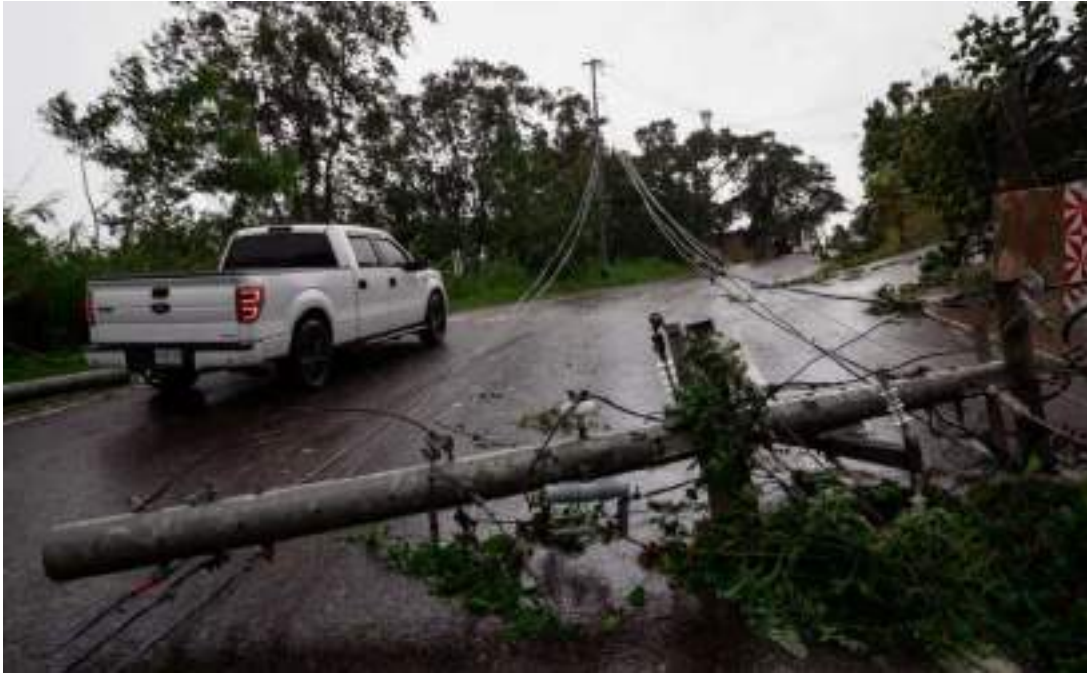
Figure 269: Photographic Evidence of Energy Infrastructure Collapse After Hurricane Fiona in Puerto Rico 992
