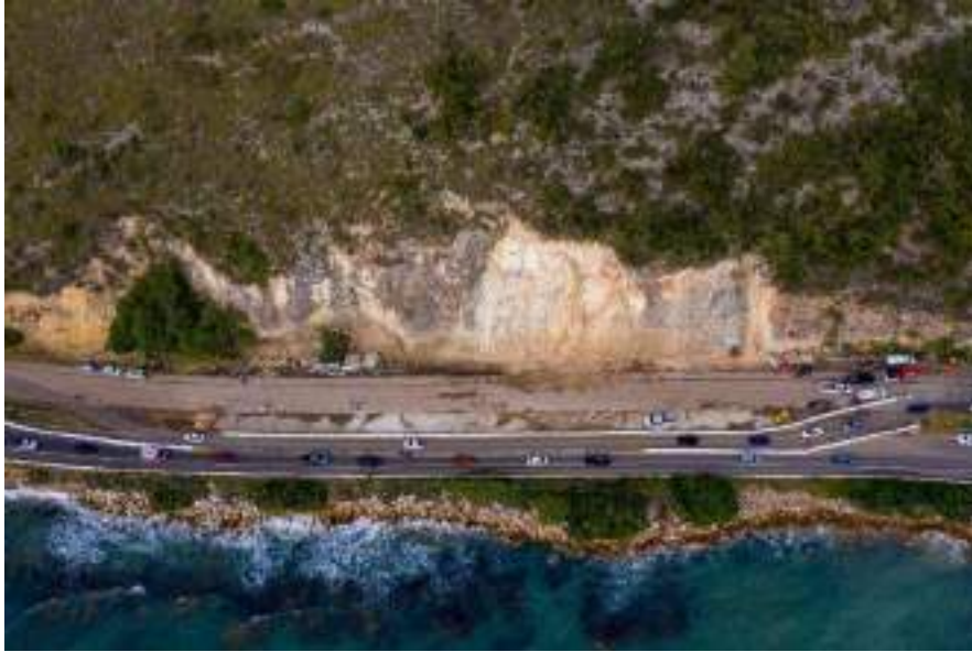
Figure 117: Cars Navigate Landslide Area After Earthquake Ponce 303
