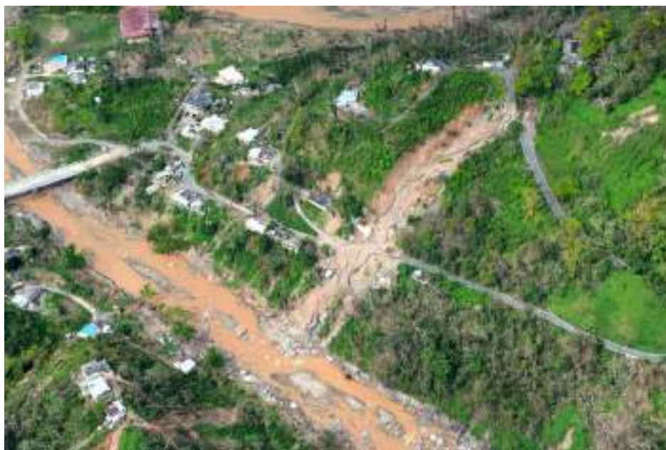
Figure 184: Landslide Along PR-4131 in Lares, Puerto Rico, 2017 648
