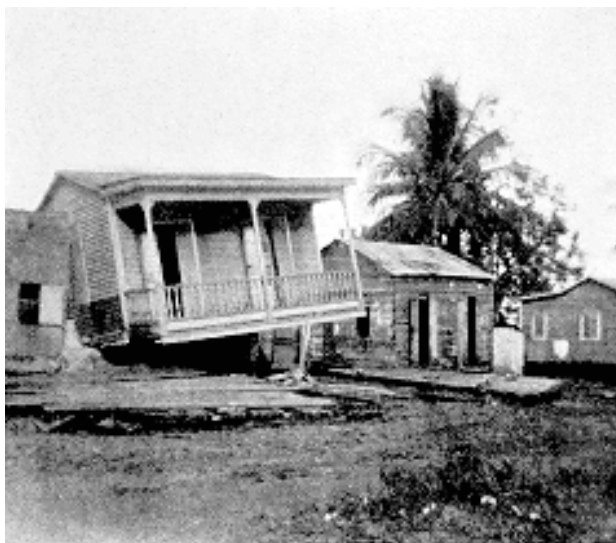
Figure 247: Subsidence from an Earthquake, 1918
