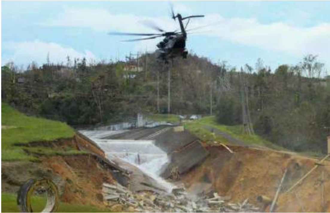
Figure 311: Damaged 54-Inch Siphon Line, Which Cut Off Water Supply to the Western Side of the Island
