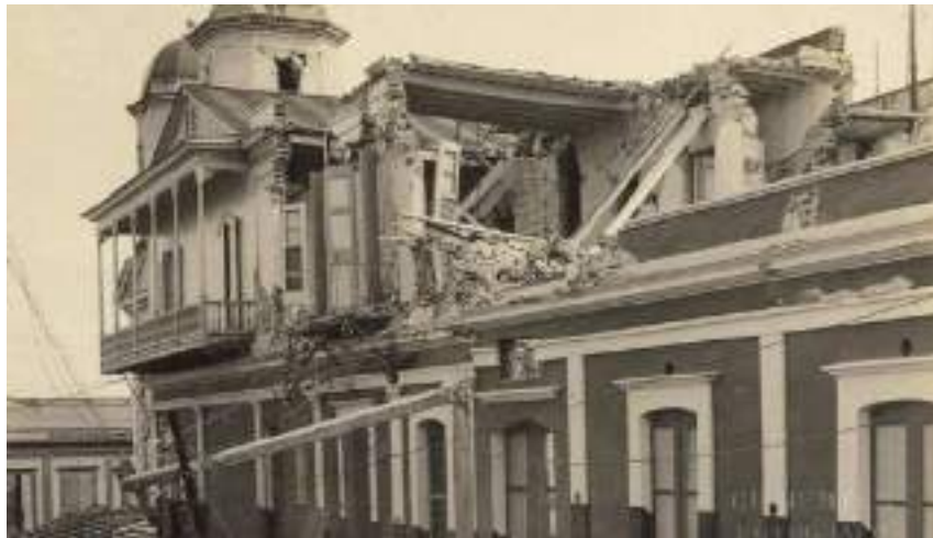
Figure 100: La Mallorquina Building Damaged by the 1918 Earthquake in Mayagüez 283
