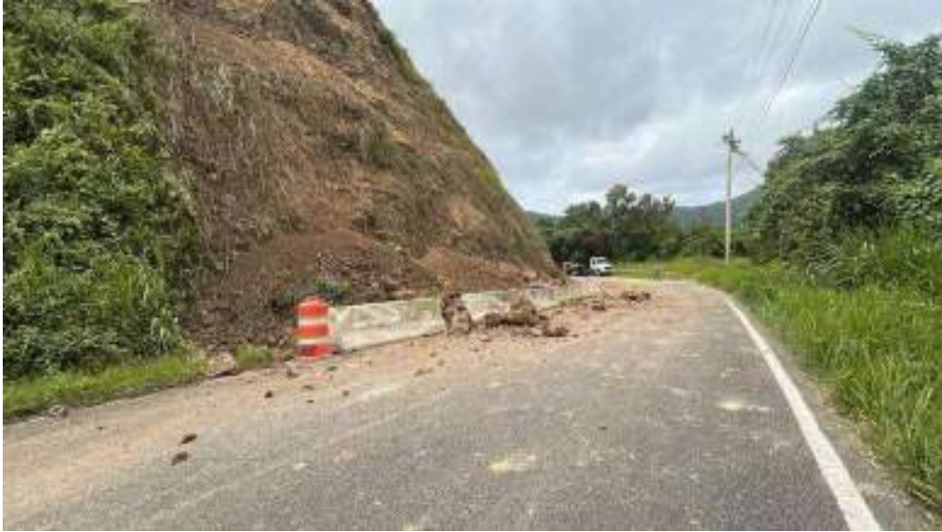
Figure 195: Landslide on Road Leading to the Carite Community in Guayama, June 19, 2025 668
