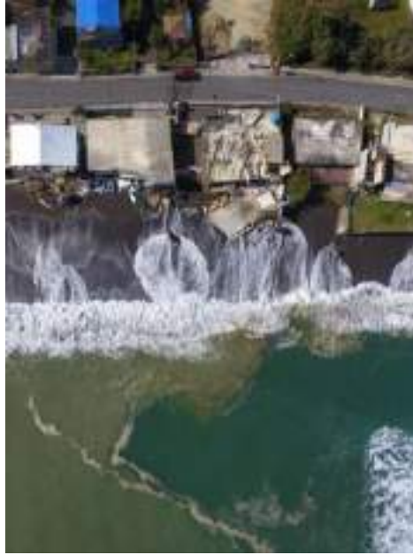
Figure 64: Coastal Damage at Playa de la Boca, Barceloneta 171
