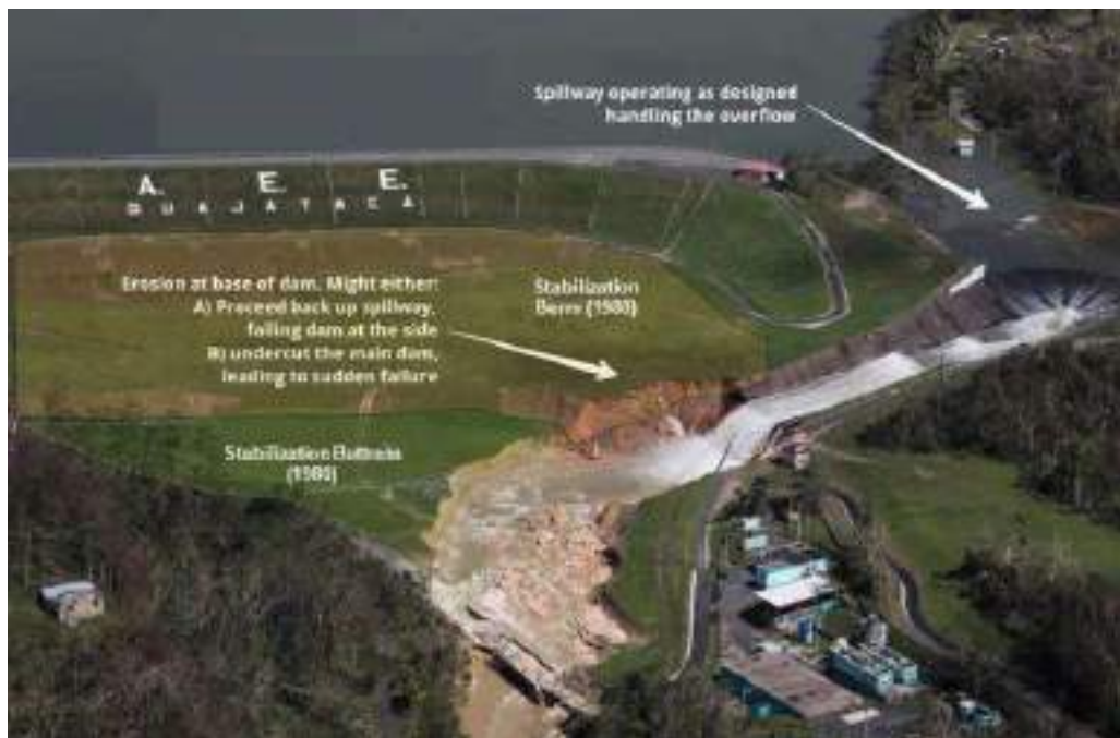
Figure 310: Damage to the Guajataca Dam Spillway Following Hurricane Maria 1156
