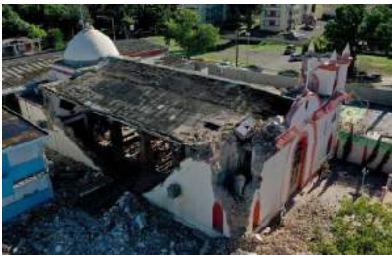
Figure 104: January 2020 Earthquake Destroyed Historic Parish in Guayanilla 290
