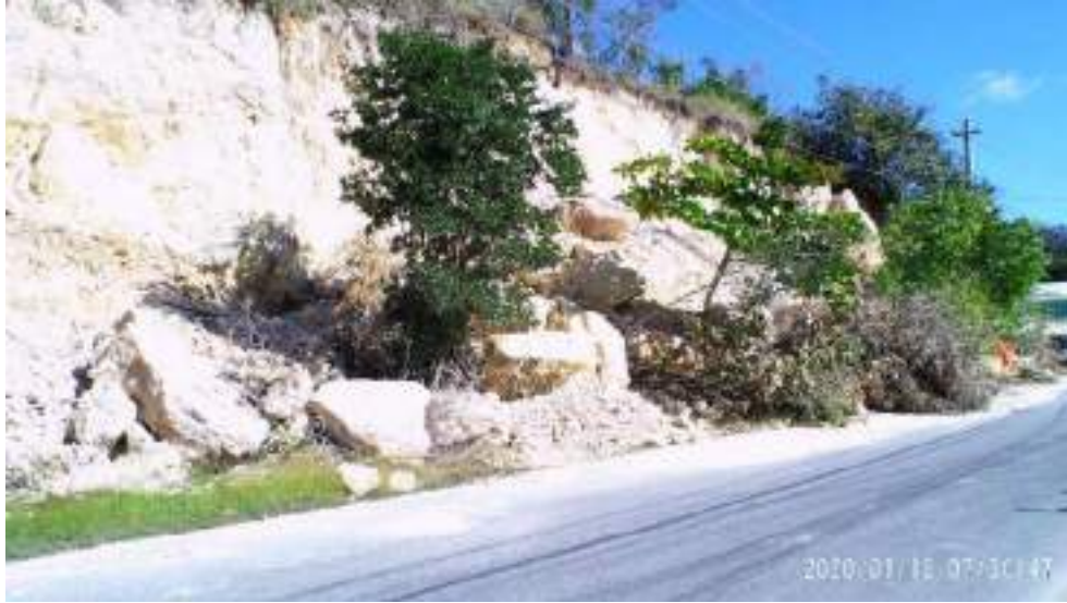
Figure 183: Landslide in Ponce, Puerto Rico, Triggered by the 2020 Earthquake 645
