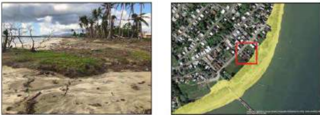
Figure 80: Ground-Level and Aerial Views of Storm-Induced Beach Erosion in Punta Santiago Following Hurricane Maria 218
