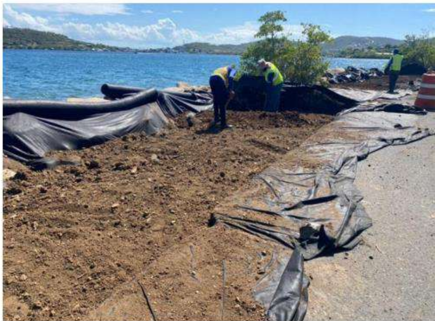
Figure 83: Installing Geotextile Fabric
