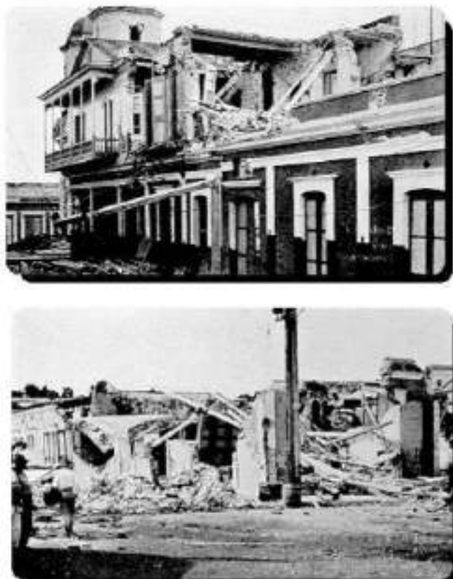
Figure 101: Damage from the October 11, 1918, San Fermín Earthquake 284
